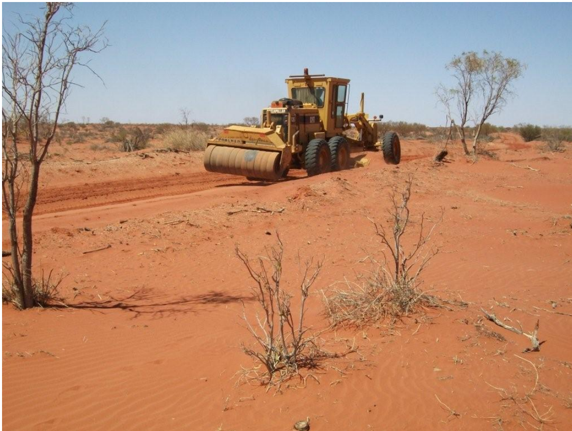
Road clearing along the Binns Track leading to CBM 107-002.
