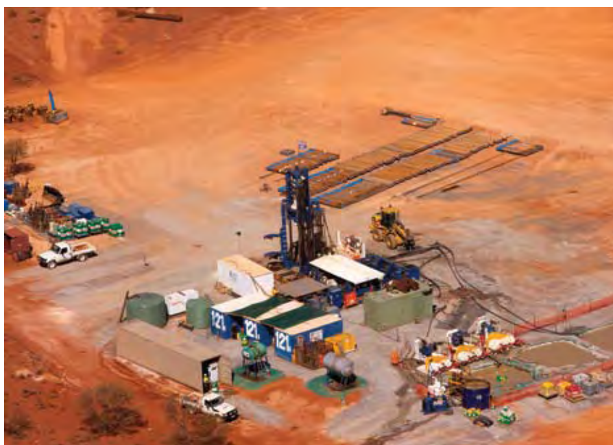
The raisebore site during reaming of the ventilation shaft
