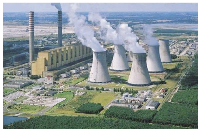
Belchatow, Poland - A third flagship project
