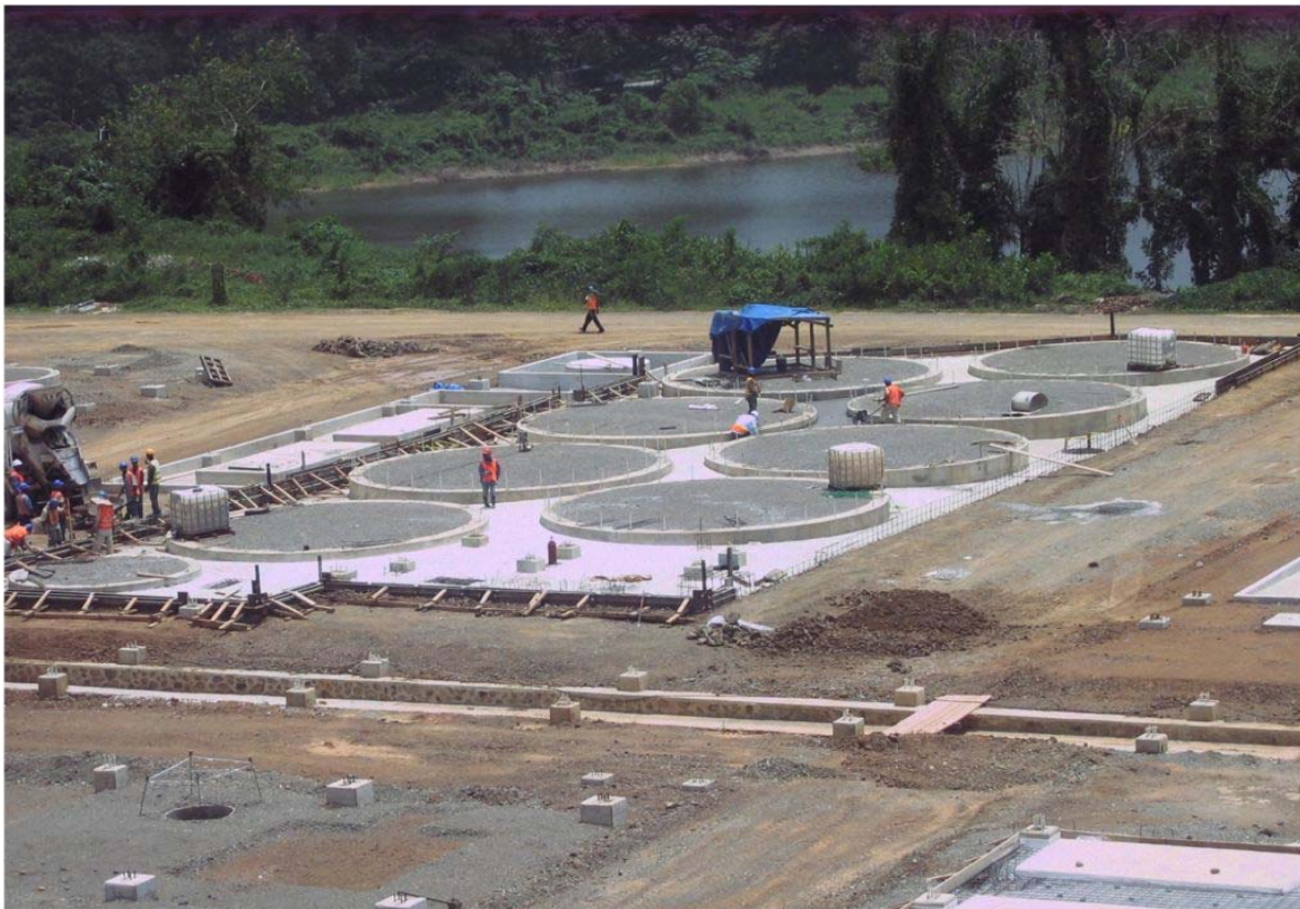
Las Lagunas Concrete Foundations and Structures
