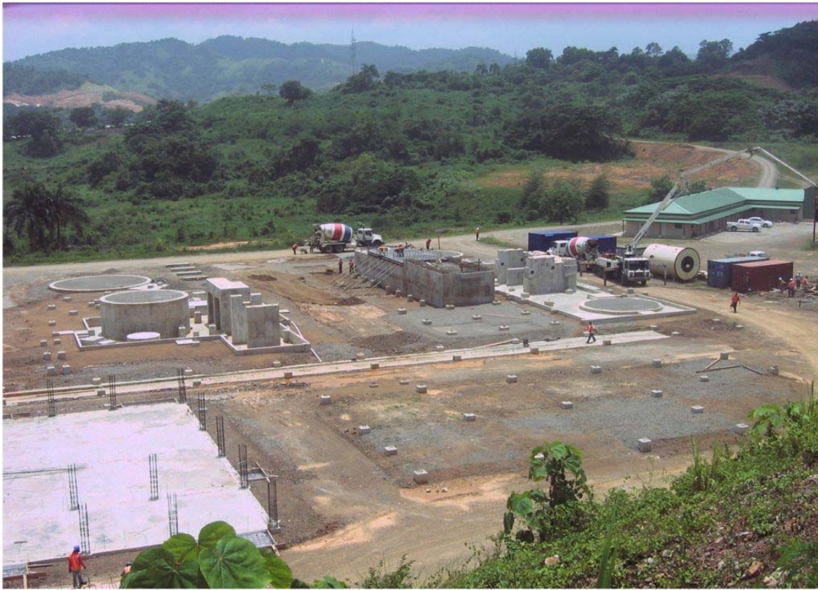
Las Lagunas Concrete Foundations and Structures
