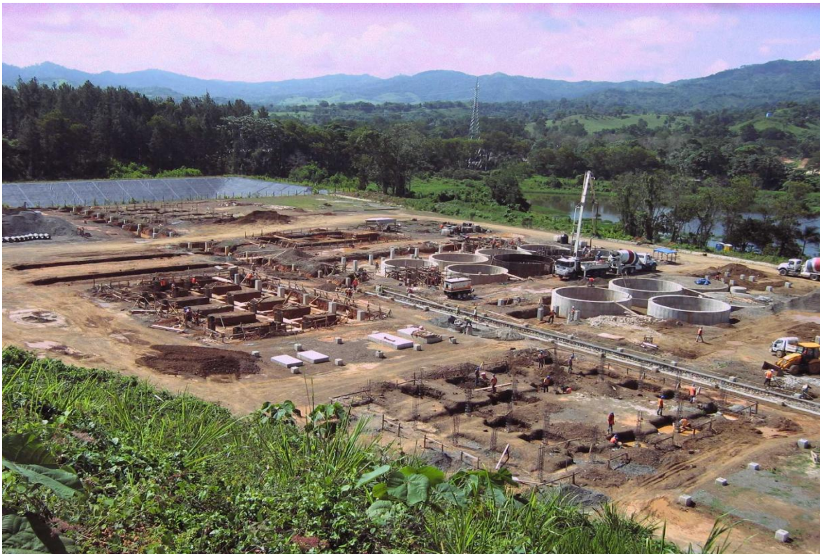
Las Lagunas Concrete Foundations and Structures
