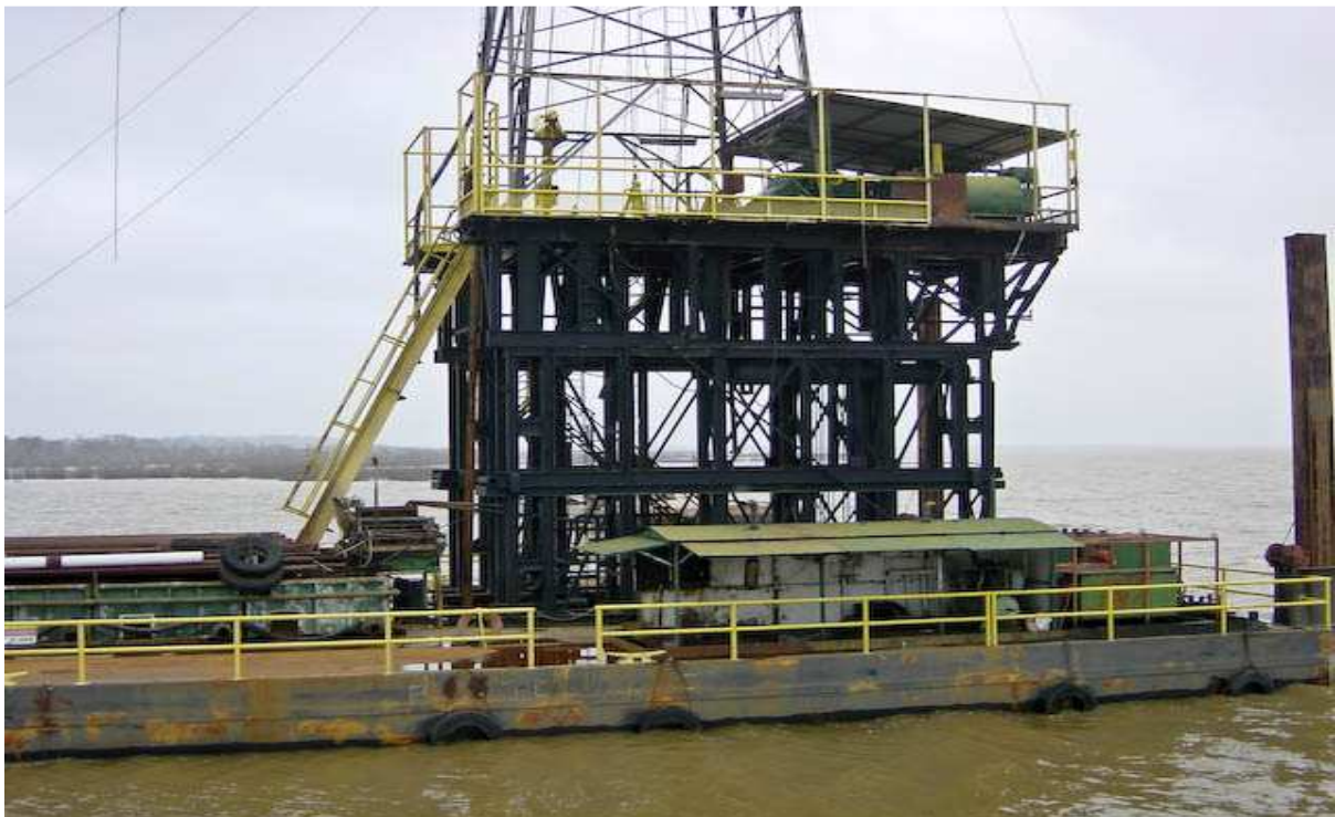
The Barge Rig
