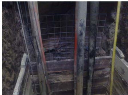
Fig 7. Services on west wall
