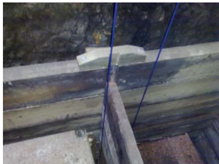
Fig 6 plumb lines for shaft refurbishment
