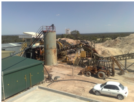
Figs 8 & 9. Leach tanks on the pad and CIP pre treatment tank
