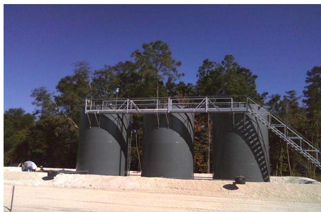
New storage facilities at Silverwood
