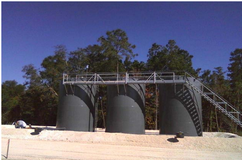
New Tank Facility at Silverwood
