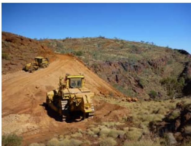
Fig.2; Mt Webber northern access ramp construction.
