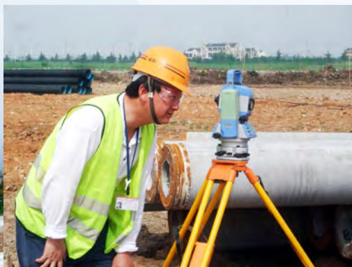
Jiangsu Surveyor Onsite
