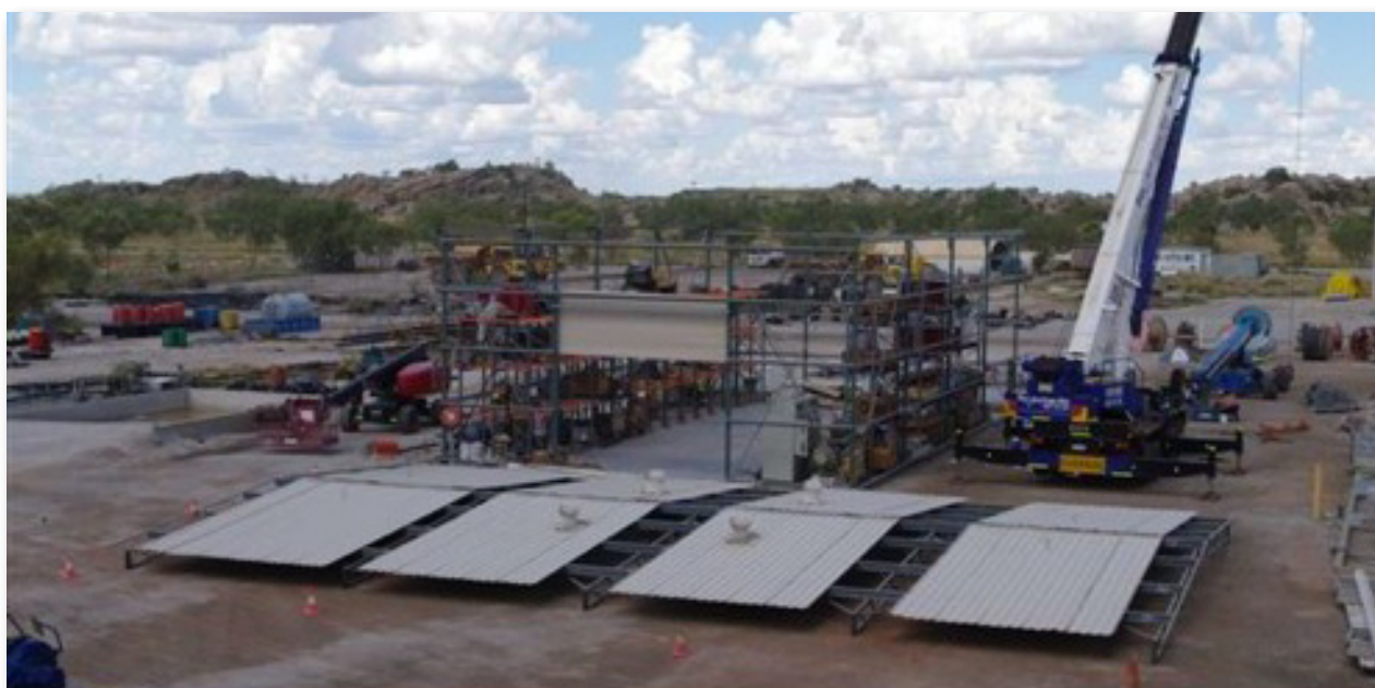
Plate 1. Flotation building roof ready for dismantling at Pillara
