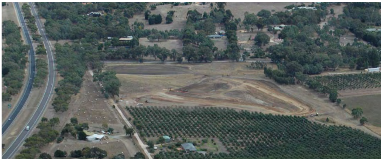
Plate 1. Brown Dam Under Construction
