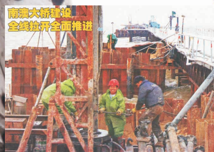
CONSTRUCTION OF BRIDGE TO RECEIVING TERMINAL
