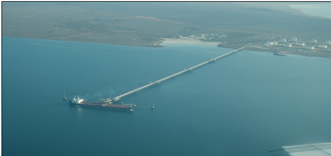
Figure 4: Aerial view of Port Bonython, showing the Santos jetty in the foreground
