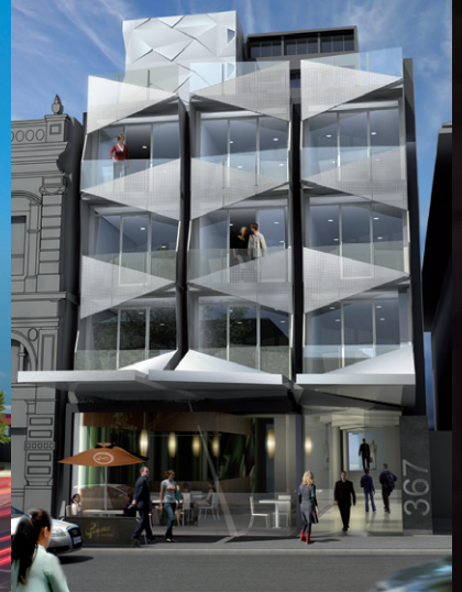
Soon to be completed - VIVIDA in Hawthorn by Tissot Developments
