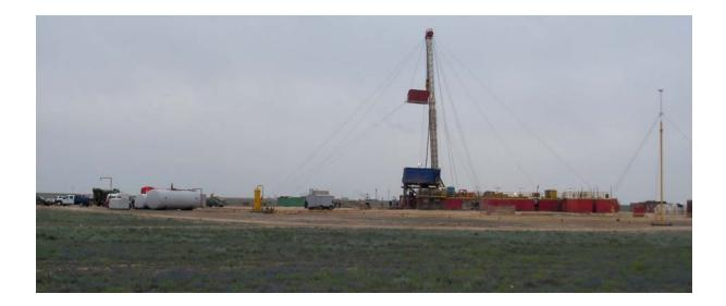
Drilling rig with the well test and temporary production spread in the foreground. Moving from right to left; the gas flare on the far right, the yellow gas-oil-water production separator in the middle left and the white discharge and buffer tanks and off-take arm for discharging oil to customer supplied tanker trucks to the left.
