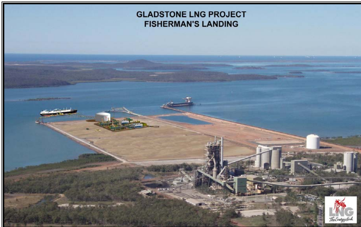
An artist's impression of the 3 mtpa Gladstone LNG Project at Fisherman's Landing.
