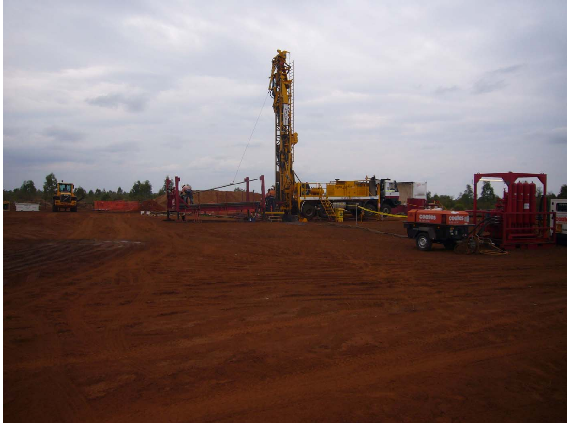
Figure 2: Working Rig – ATP 1020
