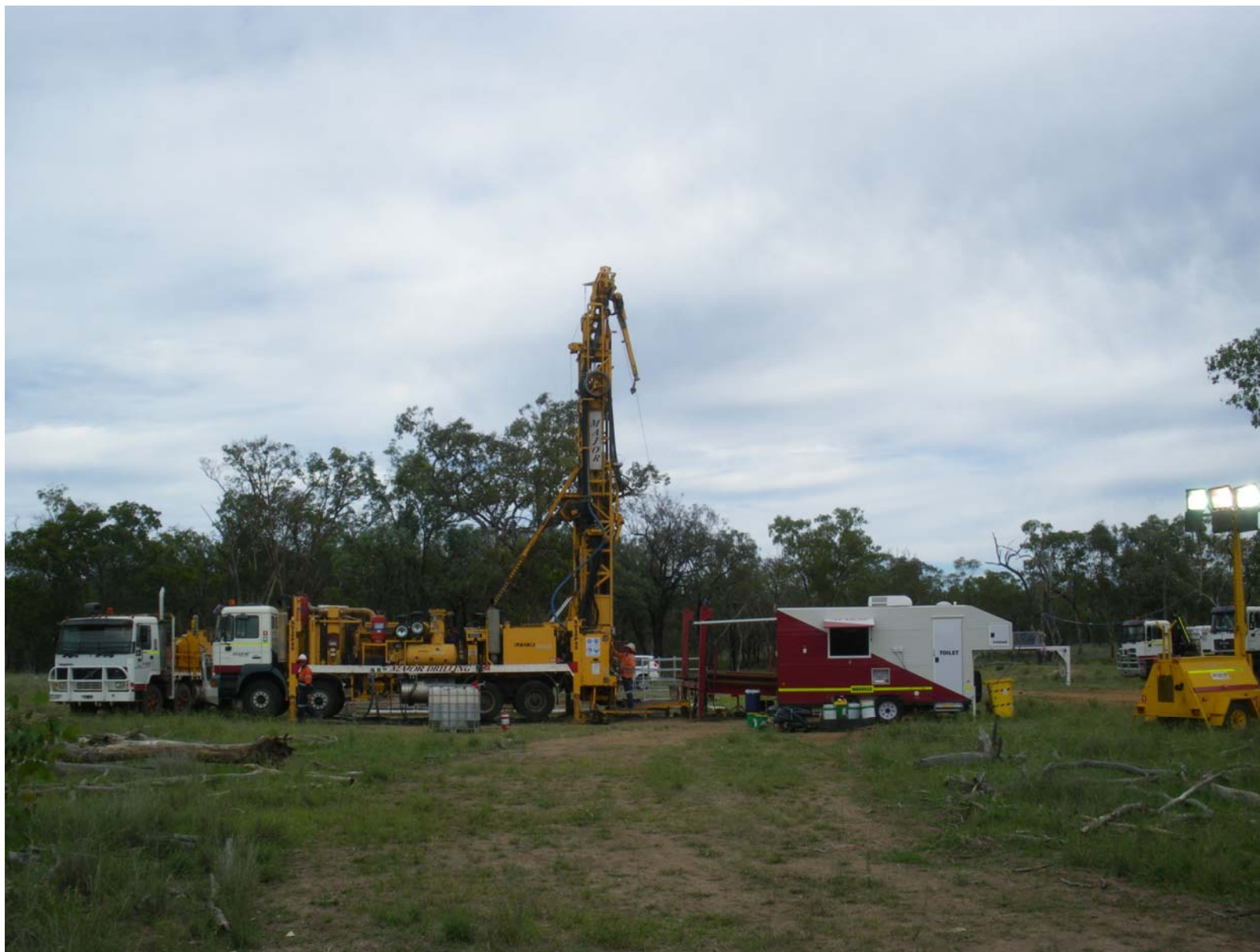
Figure 3: Working Rig – EPC 1623
