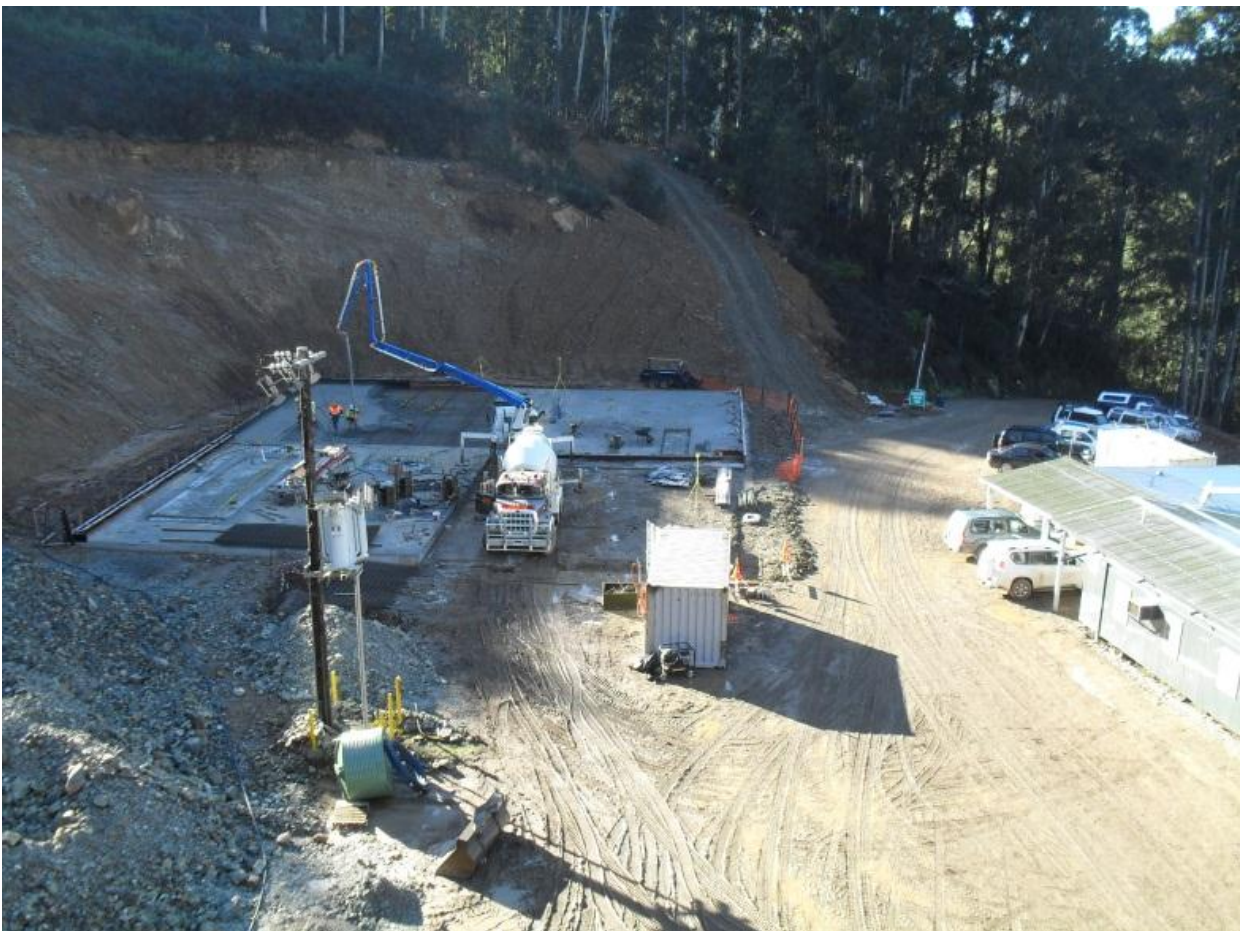
Concrete Pours at the Morning Star GPP in the Sept 2010 Quarter
