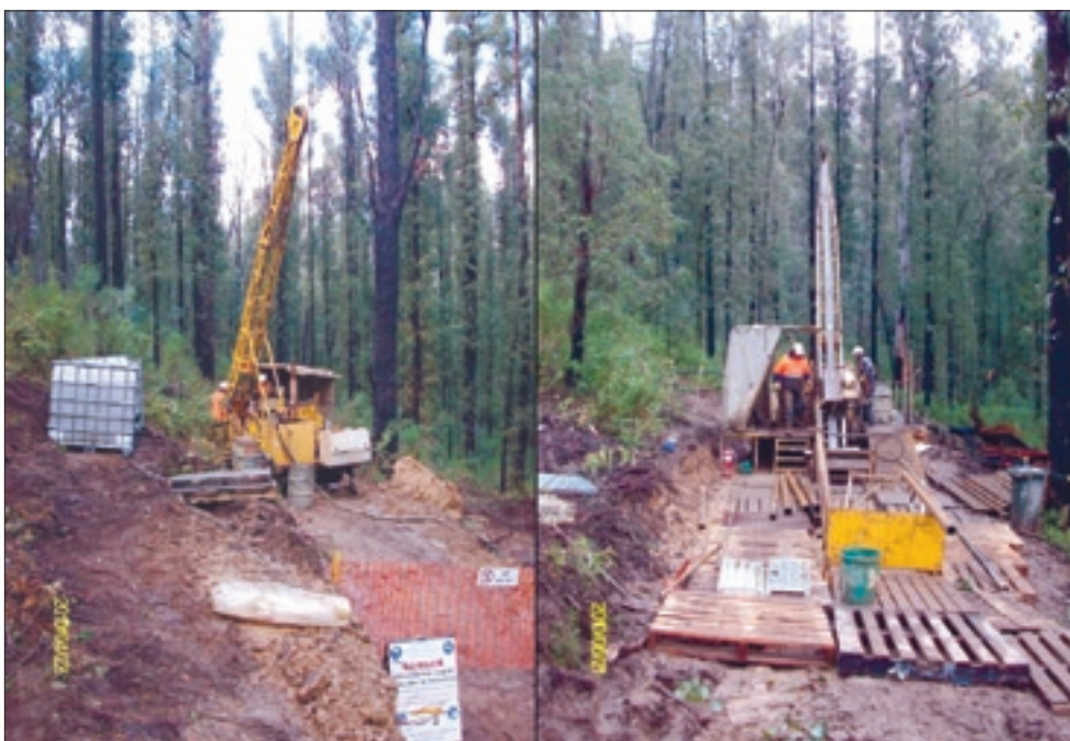
Figure 21: Drill rig set over drill hole HSD12 (LHS) and drill hole HSD13 (RHS) at Anomaly 4.
