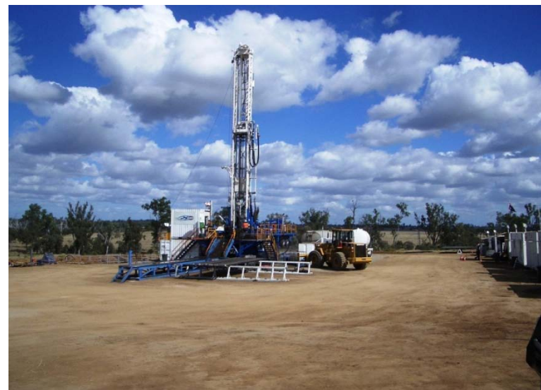
Queensland drilling operations
