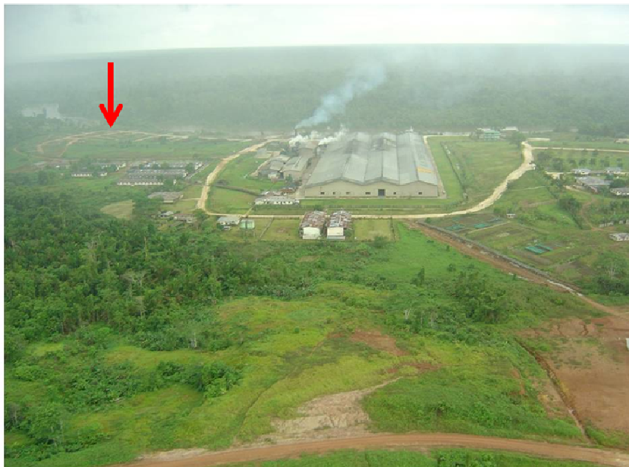
Panakawa-1 proposed well location (red arrow) in log yard of the Rimbunan Hijau Plywood Mill (view to south). Well pad construction is currently underway with heavy equipment on location. Note Wawoi River adjacent to site provides access to barges up to 3000 tons.
