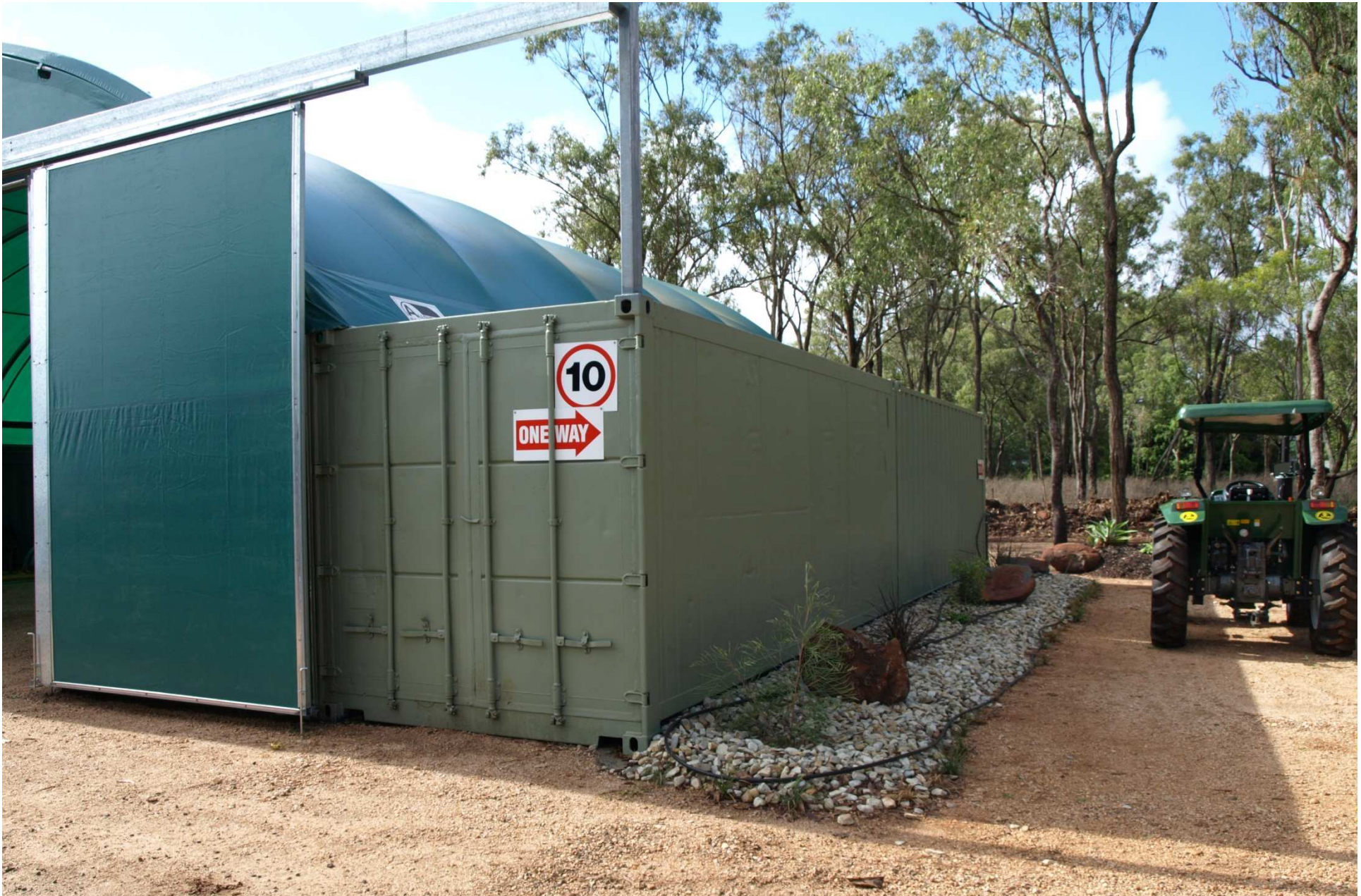
WALKAMIN FACTORY SOUTHERN SIDE CLIMATE CONTROLLED PRODUCT STORAGE SHED IN PLACE
