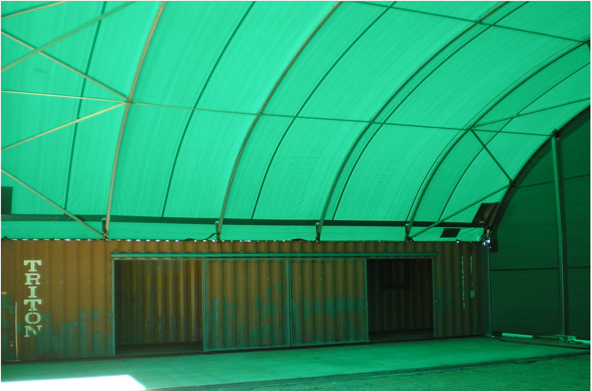
WALKAMIN FACTORY SOUTHERN SIDE MECHANICAL WORKSHOP WORK IN PROGRESS
