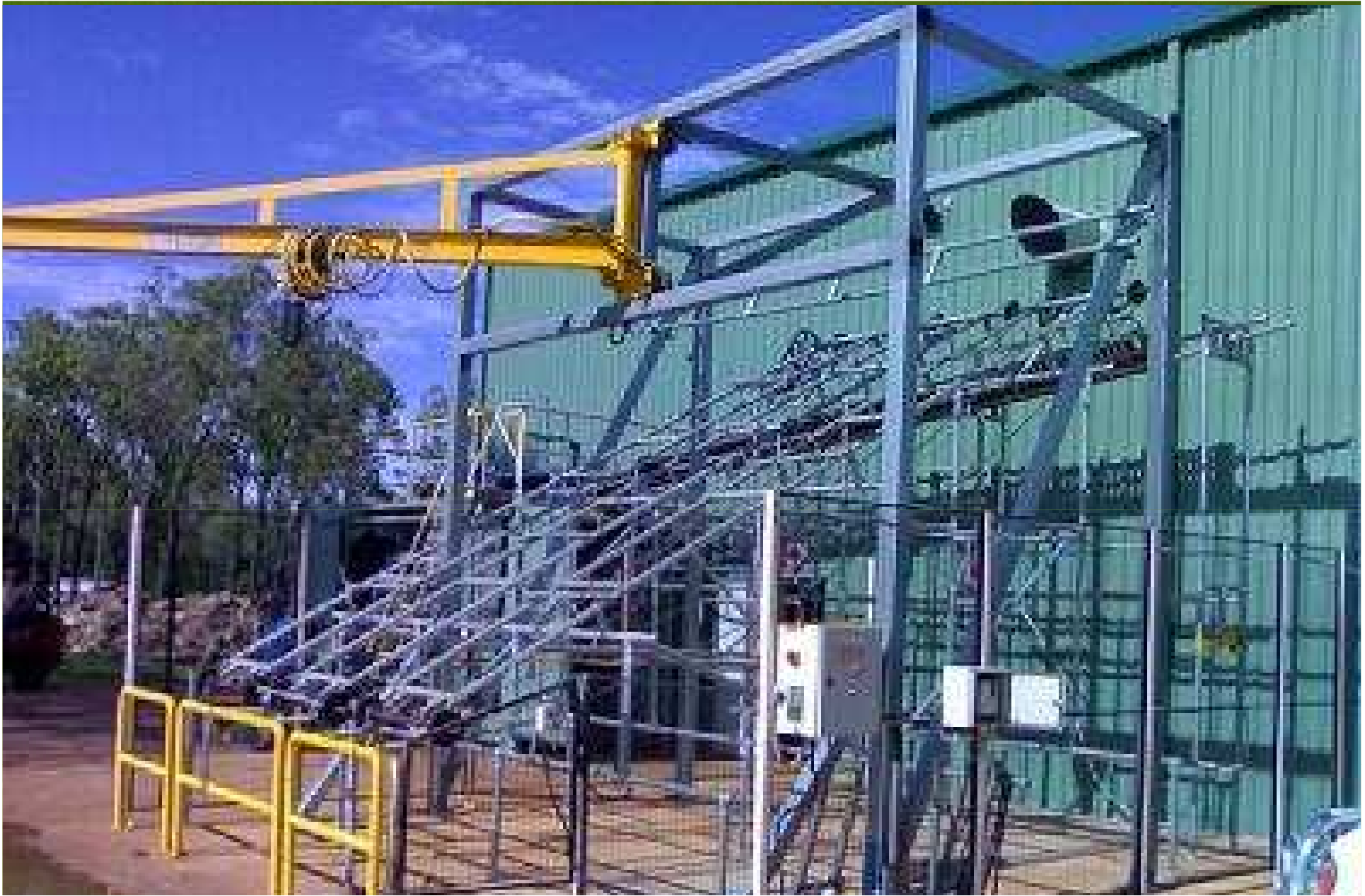
WALKAMIN FACTORY EASTERN SIDE OLD LOG YARD
