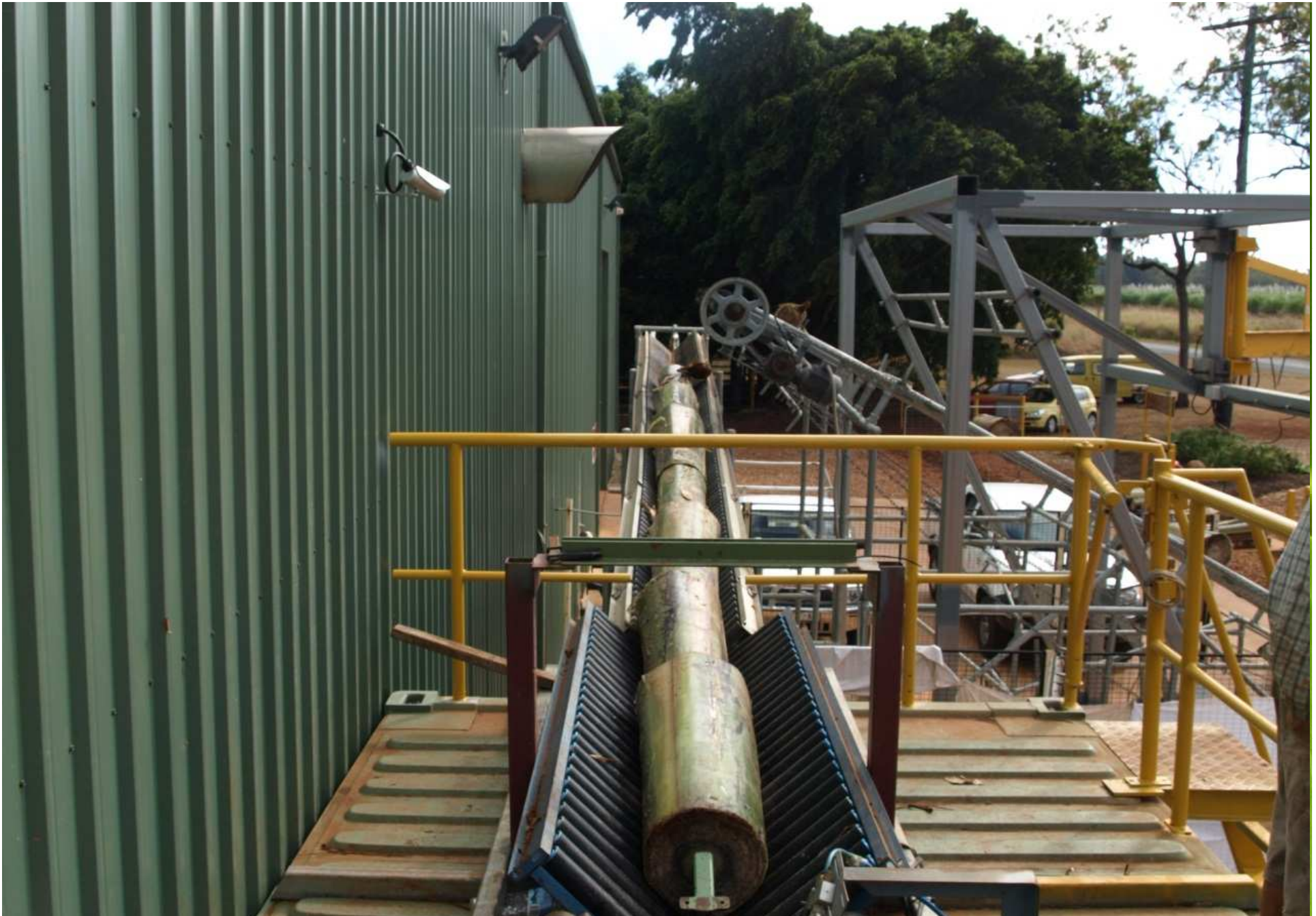
BILLETS IN THE OLD QUEUE AND DISPENSER SYSTEM
