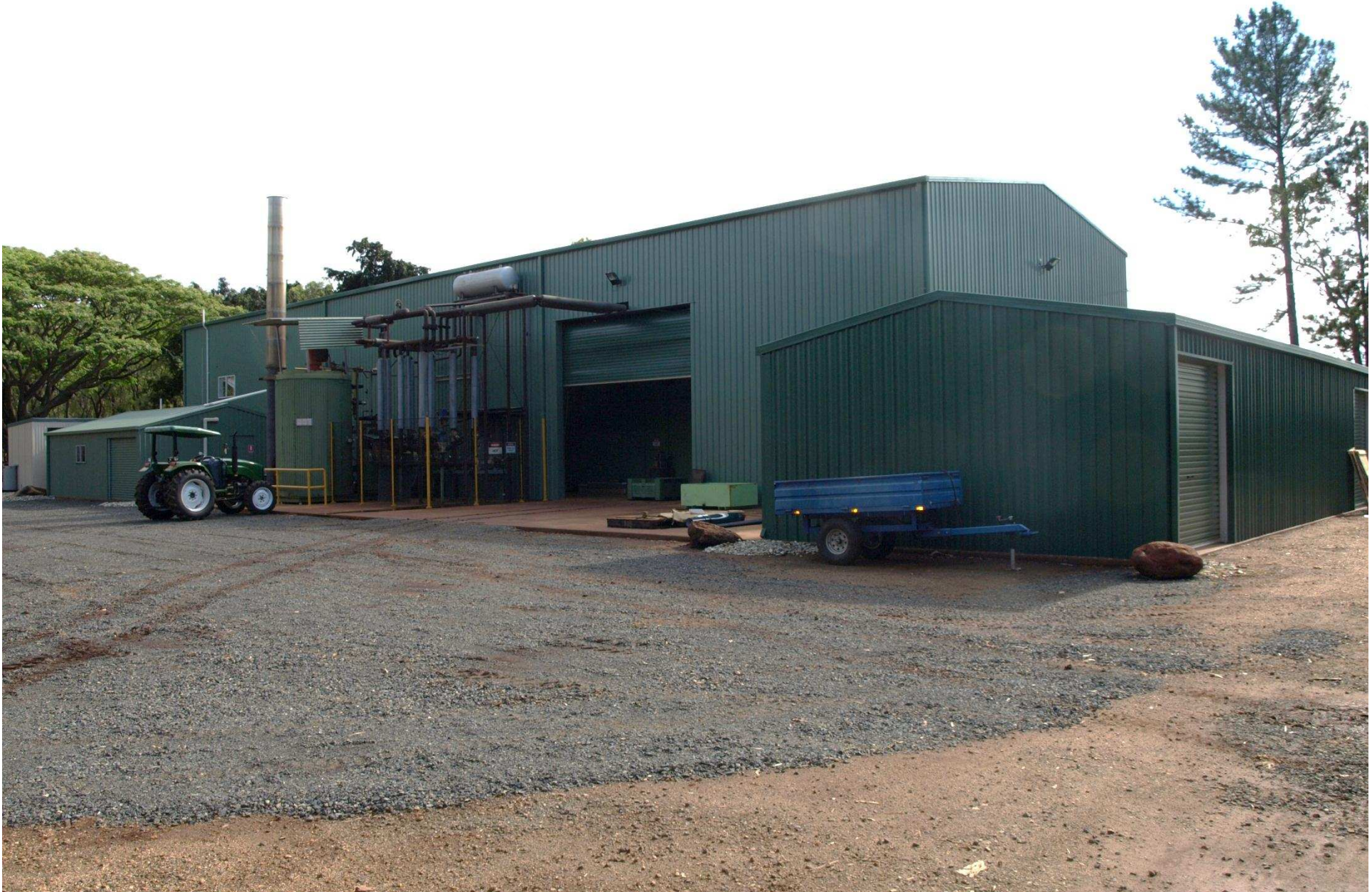
WALKAMIN FACTORY WESTERN SIDE
