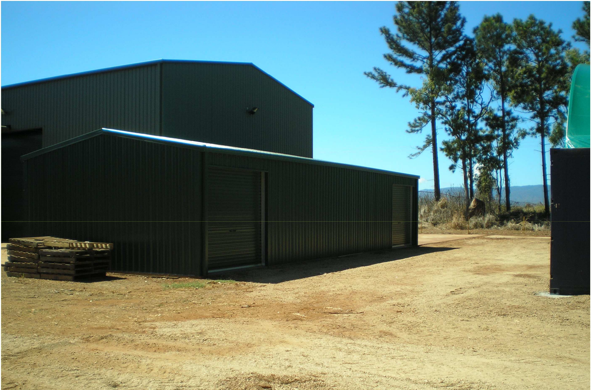
WALKAMIN FACTORY SOUTHERN SIDE PANEL PRODUCTION SHED IN PLACE
