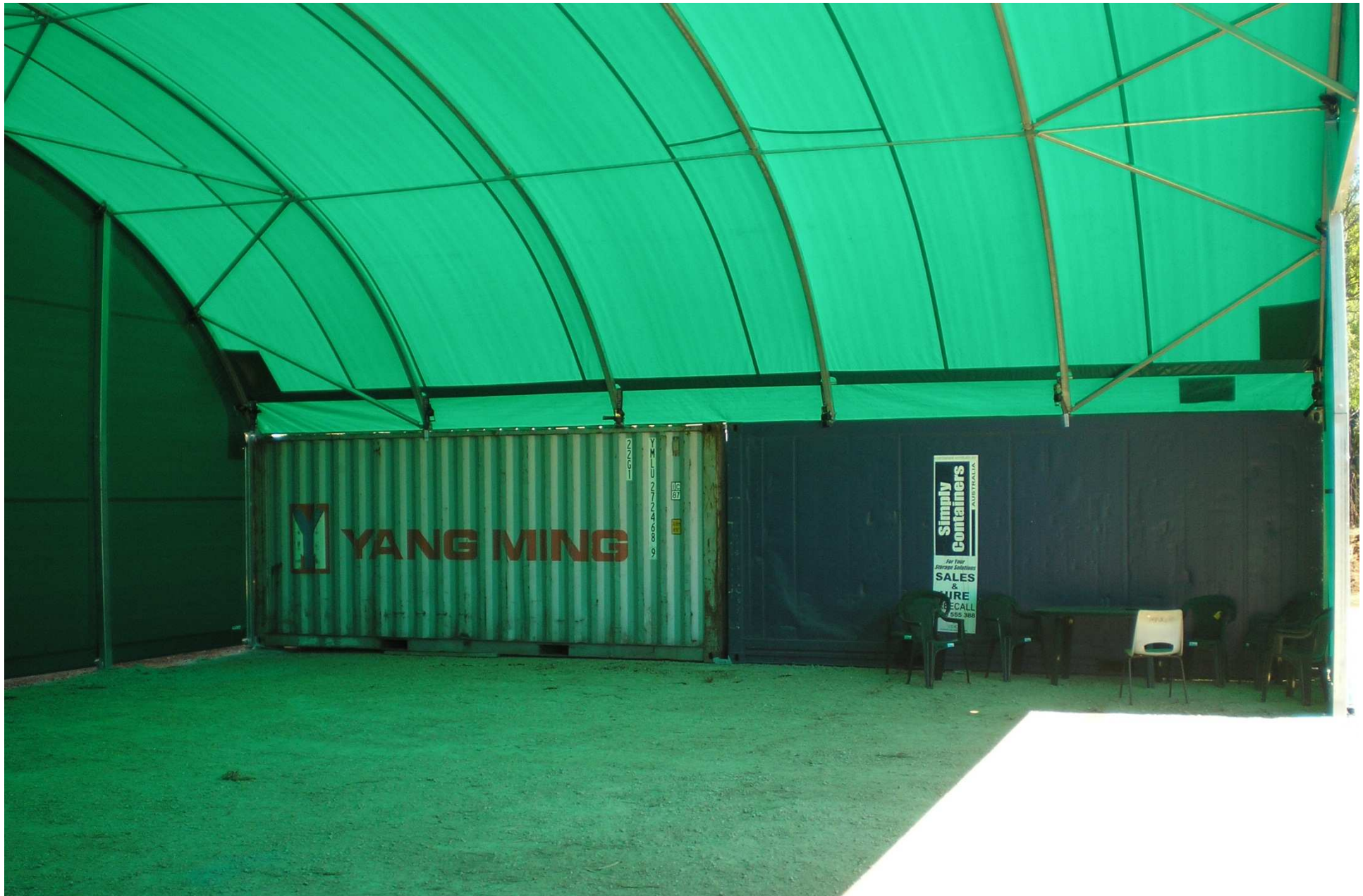
WALKAMIN FACTORY SOUTHERN SIDE CLIMATE CONTROLLED PRODUCT STORAGE WORK IN PROGRESS
