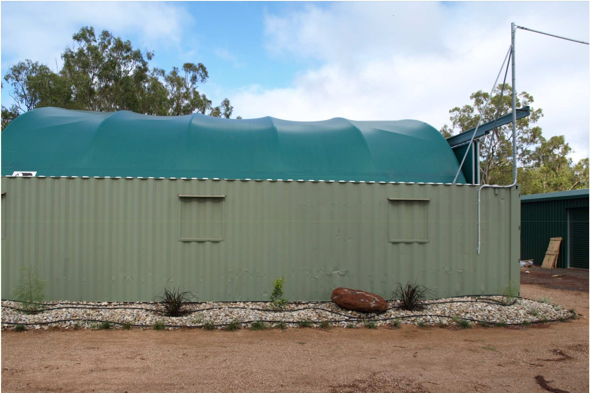
WALKAMIN FACTORY SOUTHERN SIDE MECHANICAL WORKSHOP IN PLACE
