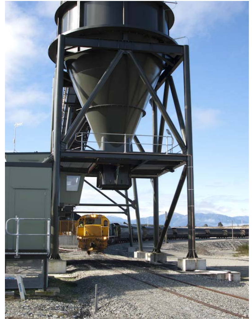
Train loading at Ikamatua
