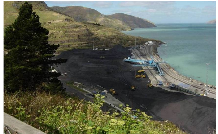
Port Lyttelton coal stockpile and handling facility
