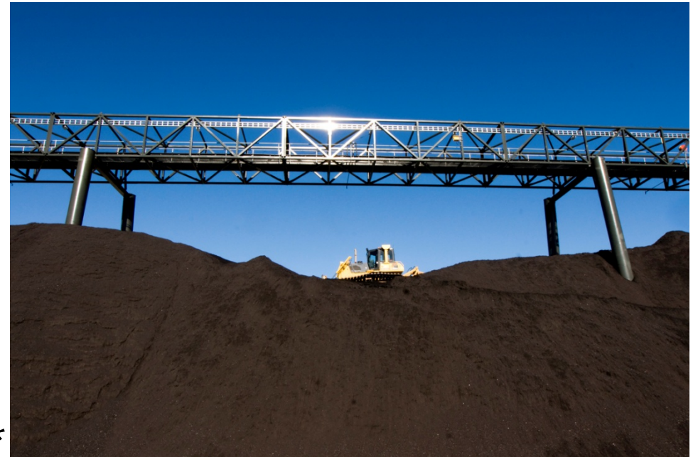
Coal stockpile at Ikamatua for second export shipment
