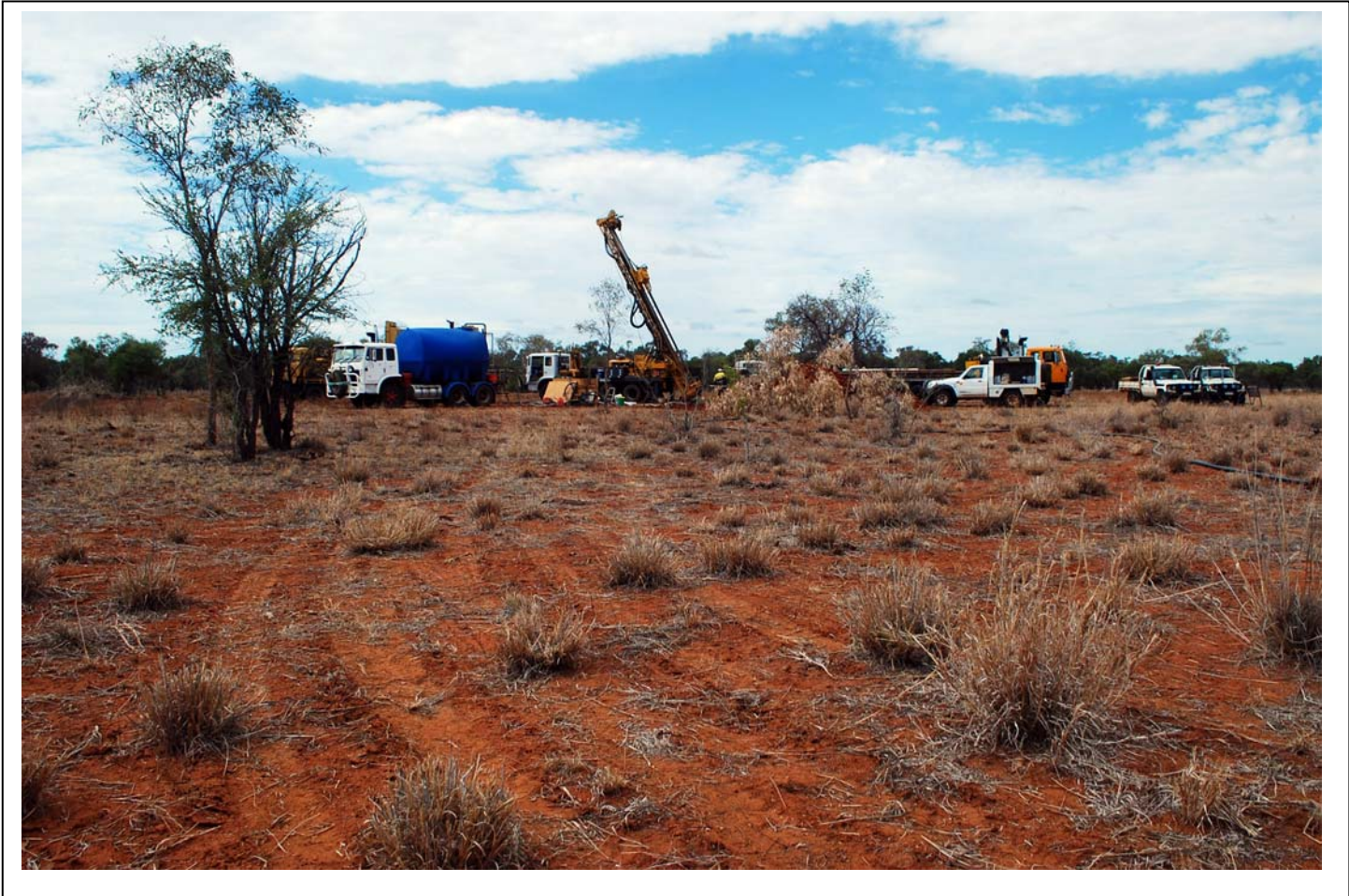
Fig. 1 Diamond drill rig operating in Jessievale
