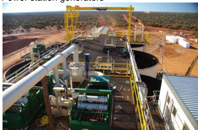
Top of CIL tanks
