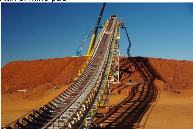
Conveyor CV1 from crushed ore stockpile
