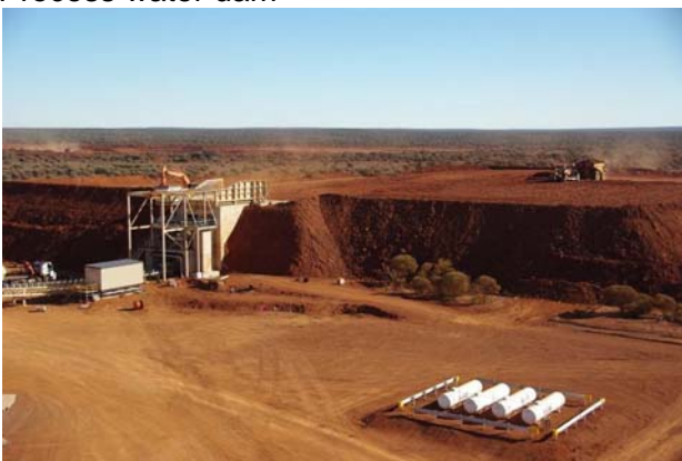
Run of mine pad
