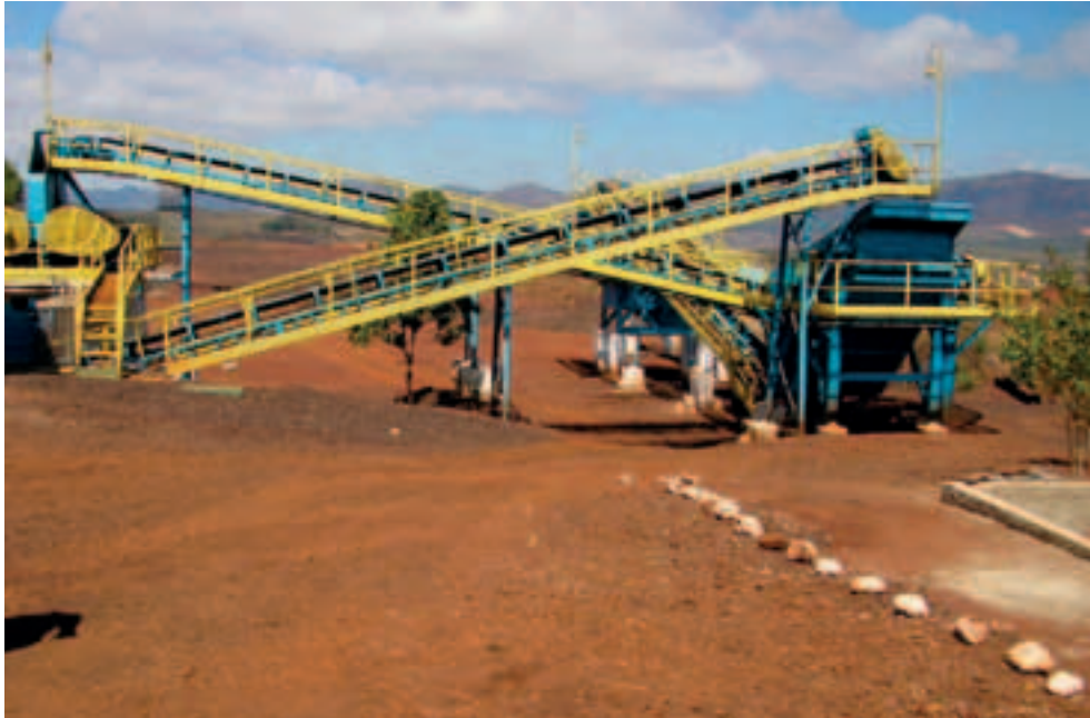
Figure 5.5_1 View across existing Ponto Verde plant
