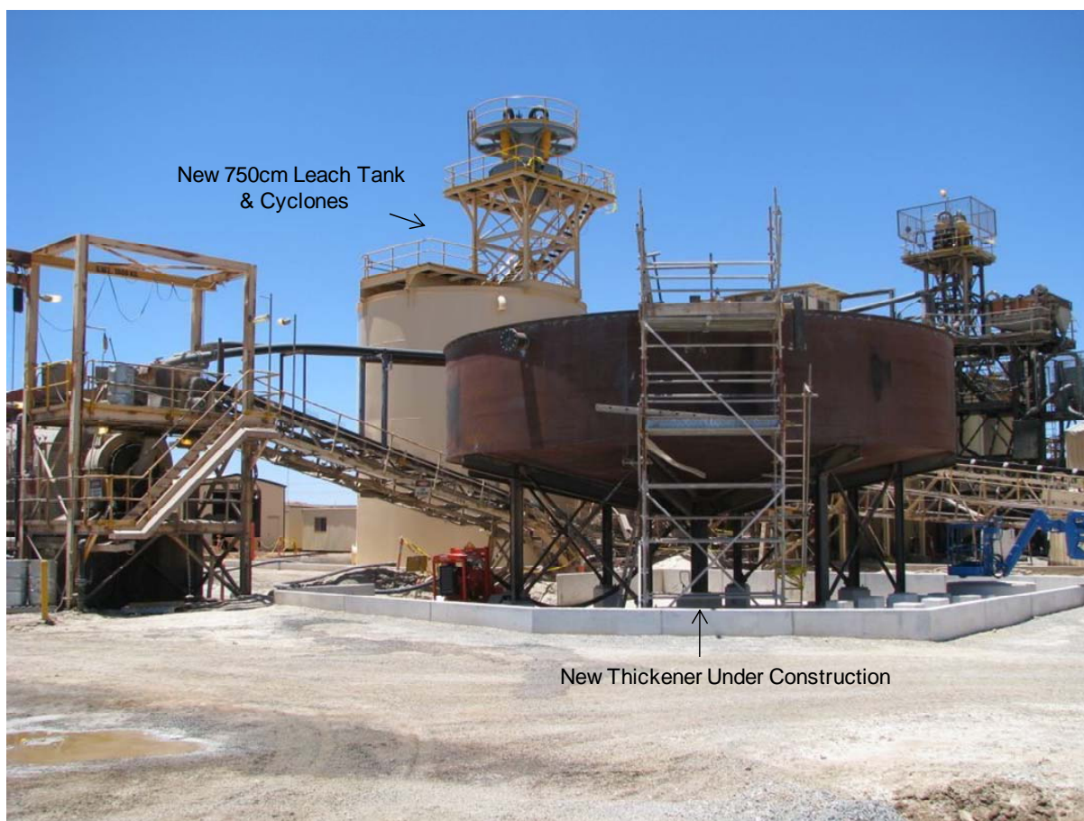
Figure 4: 600,000 tpa upgrade in progress at LGPF.
