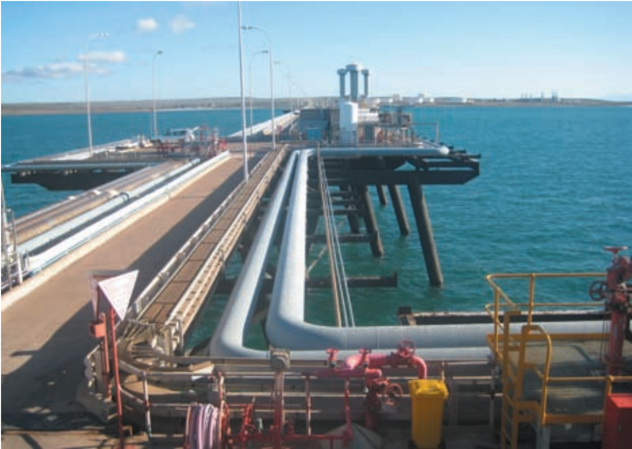
Port Bonython Jetty looking landward towards facilities which adjoin Stuart's Fuels Terminal site
