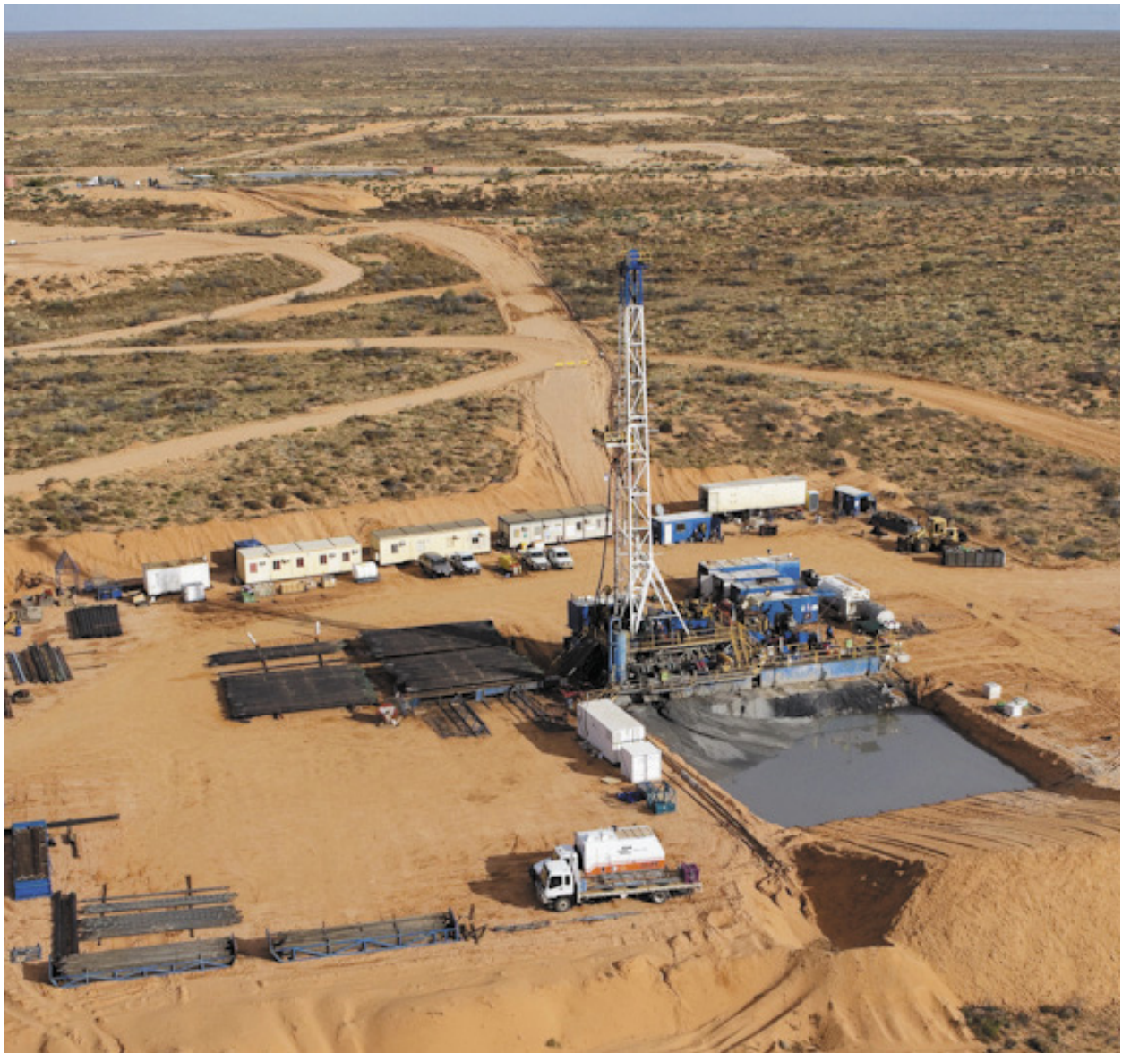
Worrior 7 oil drilling rig, Cooper Basin, with the Worrior facilities in the background
