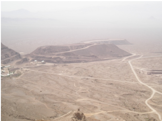
Mehdiabad Project waste stockpile and pre-strip of East Ridge
