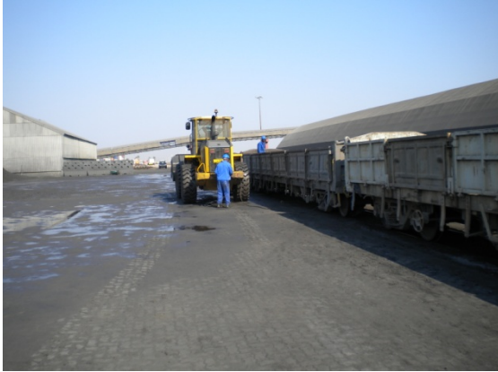
Port loading facilities at Walvis Bay, Namibia
