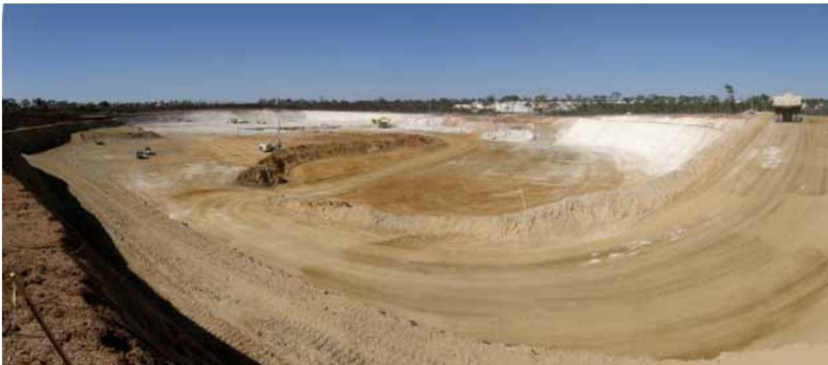
Figure 1: Spotted Quoll Pit showing weathered granite (white) overlying host mine sequence
