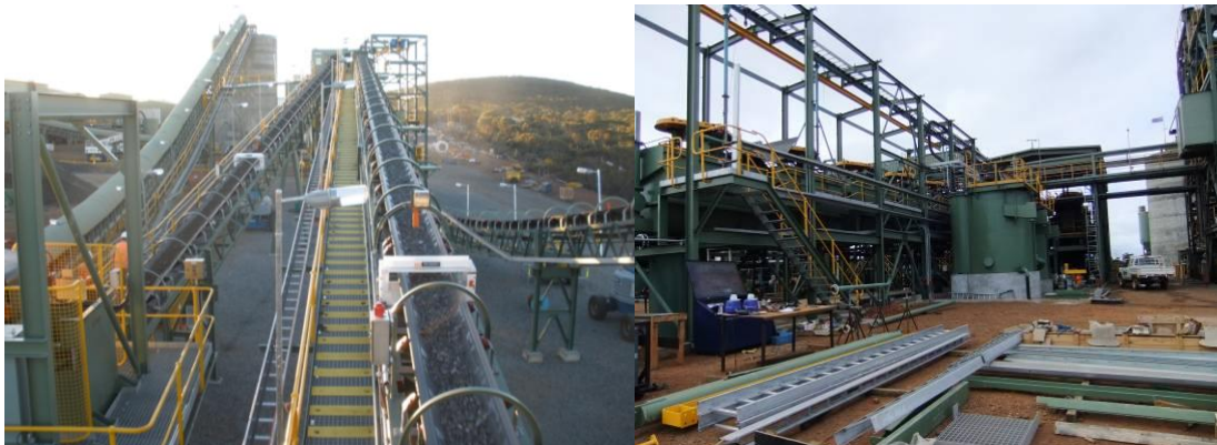
First ore through the upgraded crushing circuit
