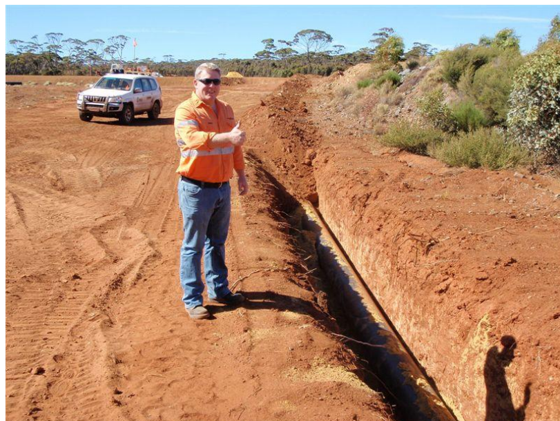
Environmental Manager Phil Knapton inspecting the dewatering pipeline at Diggers South
