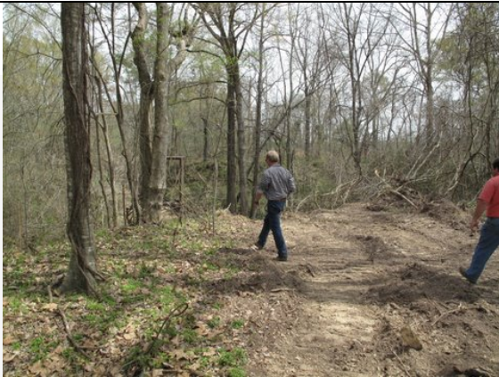
Clearing of Delivery Line Right of Way
