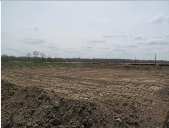
Oil Storage and Separator Pad Site Prep
