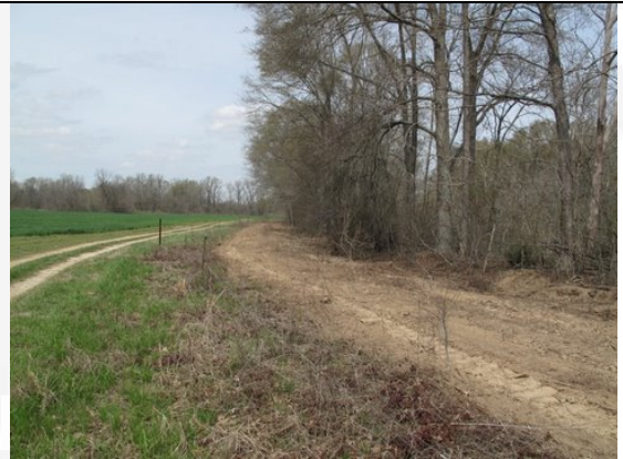
Clearing of Delivery Line Right of Way
