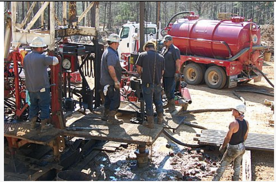
Crewmen Ready to Perforate Pay Zone
