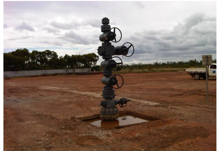
Injection well - Silver Springs 12
