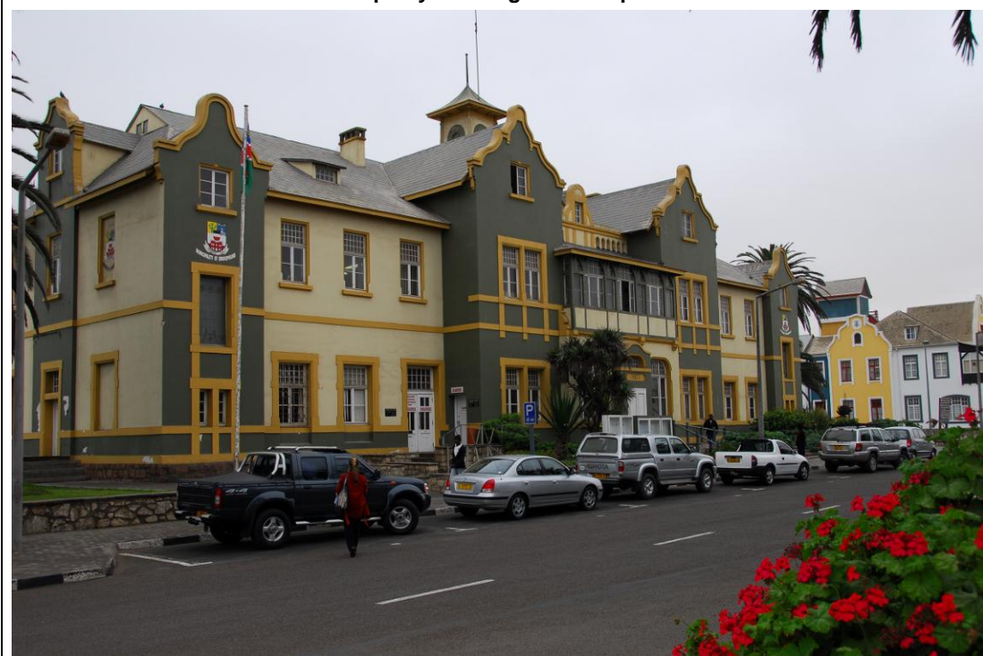
Figure 5-4 Etango Project Municipality Building In Swakopmund
