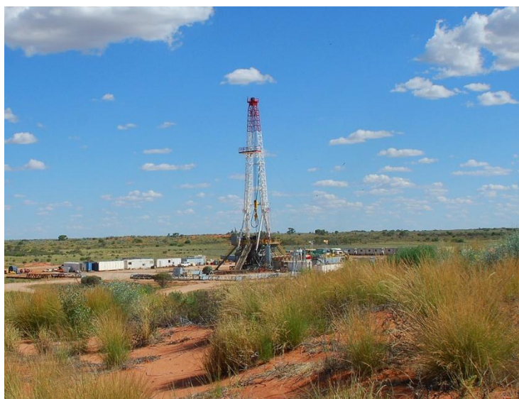
The Ensign#16 rig drilling Encounter-1
