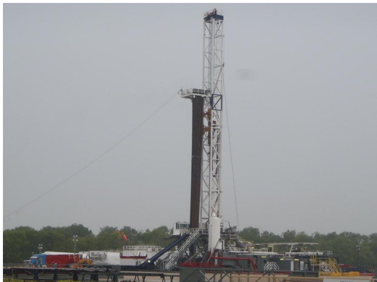
An ADR1500 rig drilling shale gas in the US
