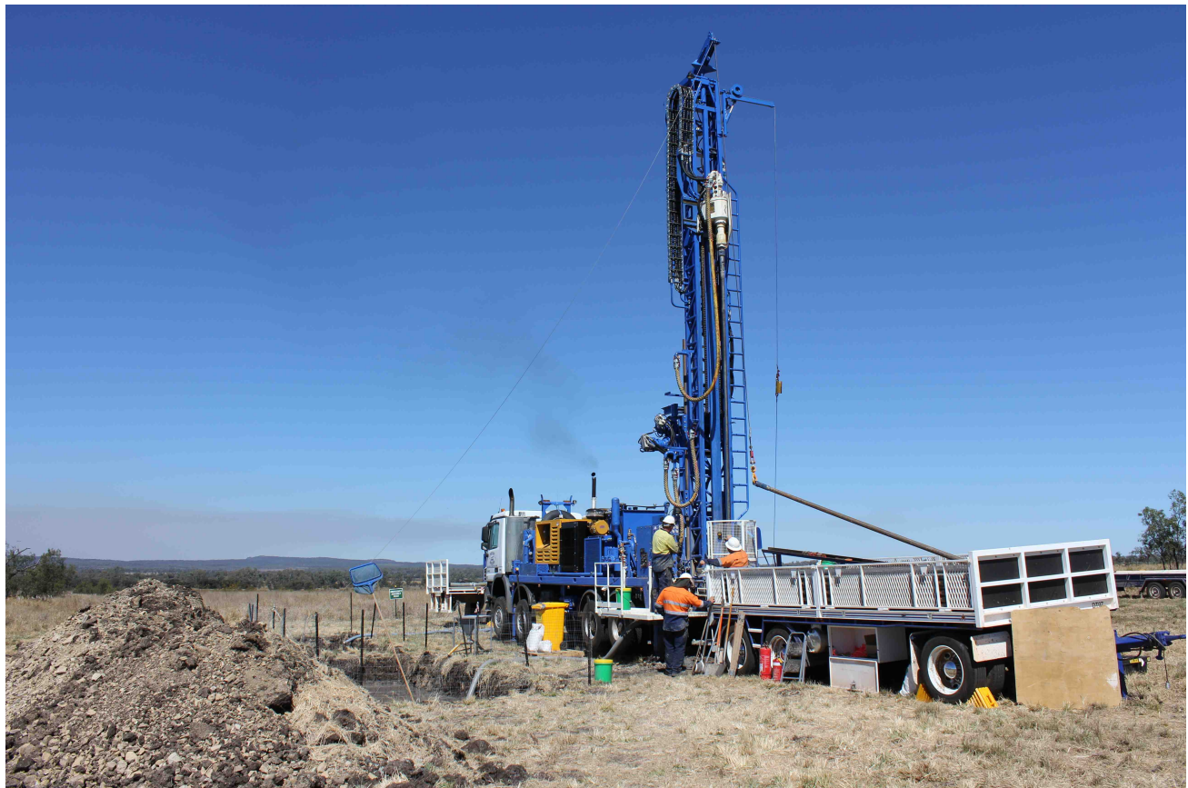
Figure 3 - South Pentland – Drilling in Progress
