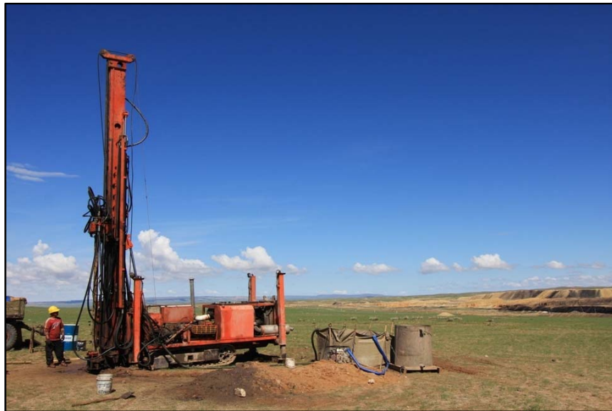
Figure 2-15: Drilling Ahead at Well Site BTE-005
