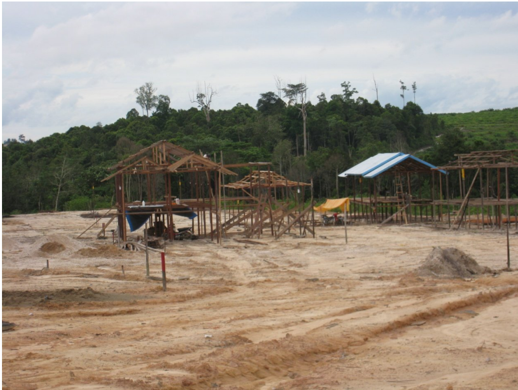
Figure 2: Construction of new houses at the new village site in progress
