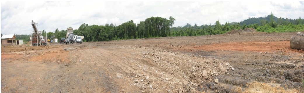
Figure 1: Completion of earthworks and crushing plant at the Abadi Stockpile
