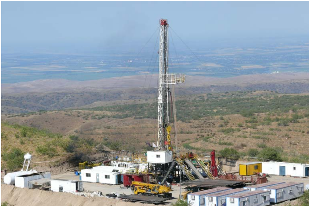
Figure 1- West Mailisu # 2 well site
