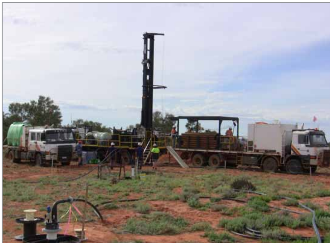
Sonic core drilling at Oban trial site
