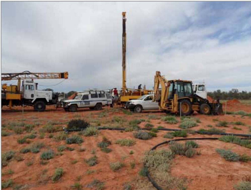
Installation of Oban leach test well field
