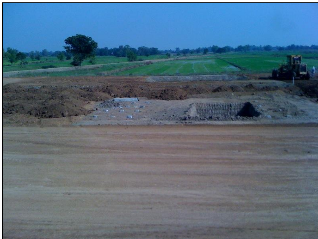
Drill site construction well advanced on Krai Thong
