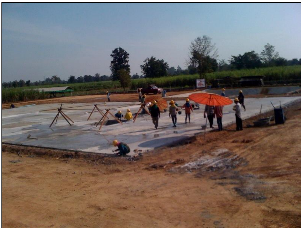
Finalising drill pad construction on Tapao Kaew as of late December 2011
