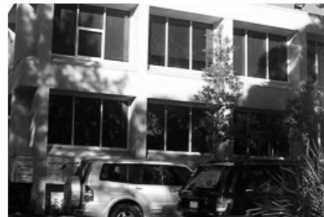
LANE COVE: 7-9 Orion Road
