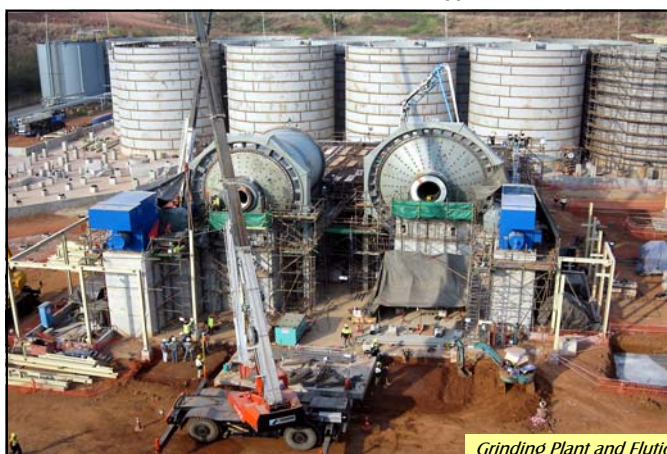
Grinding Plant and Elution Tanks under construction
