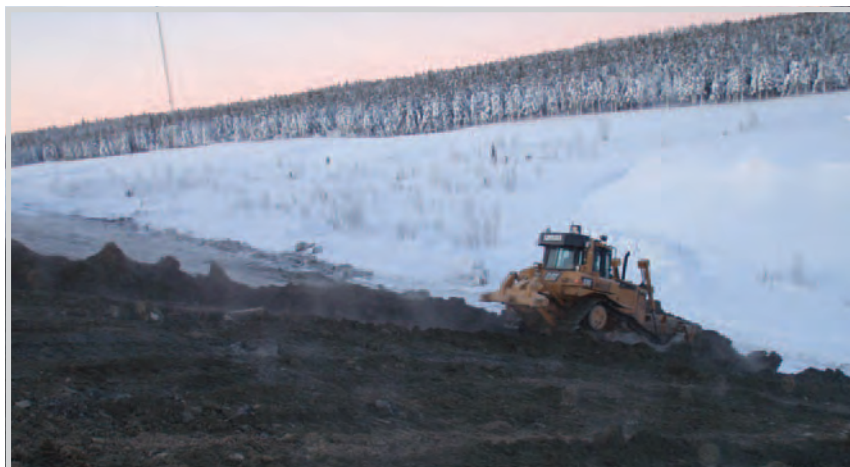
The western part of the waste rock storage facility being covered by till
