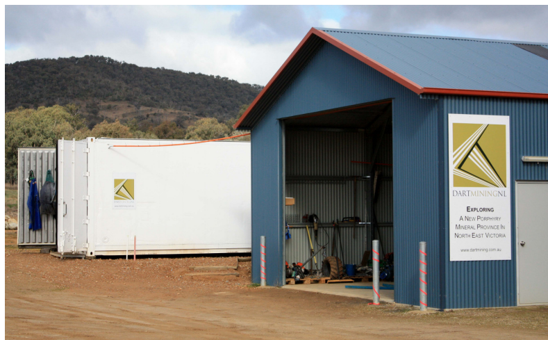
Photograph 6. New core storage shed leased from the Towong Shire Council allows rapid retrieval of stored core and assay samples required during the resource estimation process.
