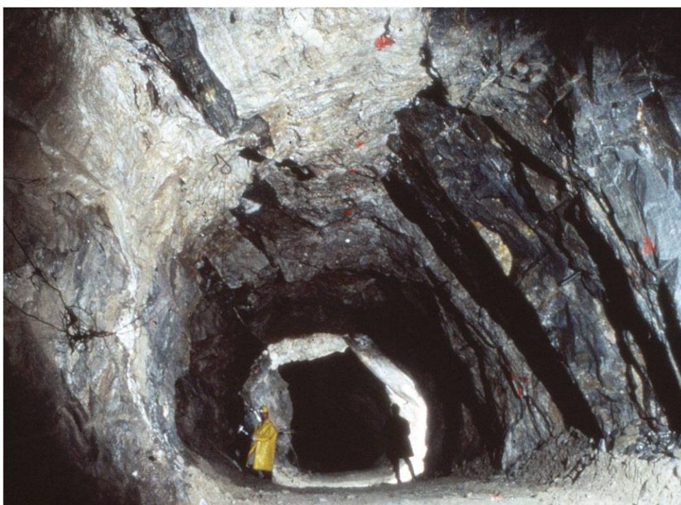
Photo 1: Ore Drive of 4 metre by 4 metre dimension
