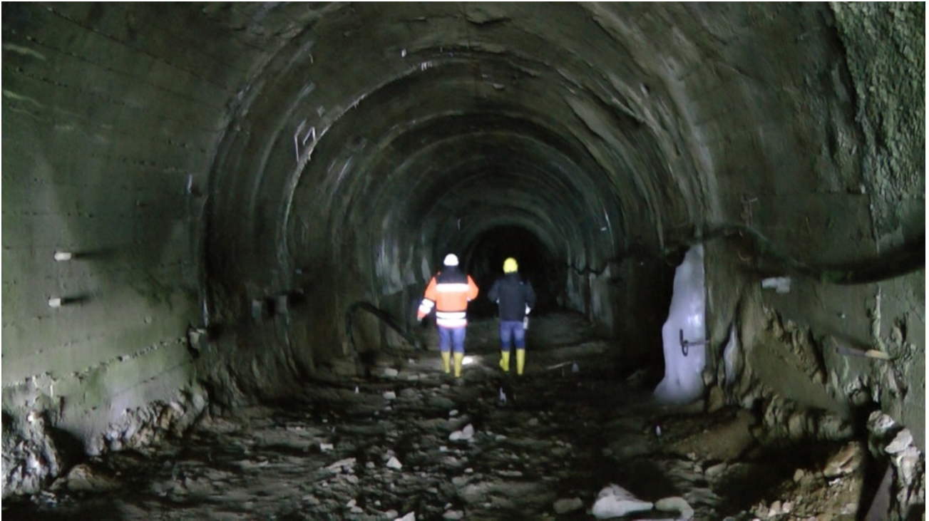
Figure 1: The decline in to the Project. Pictured is the Austrian Lithium Project Mine Manager and East Coast Executive Director Tony Roberts walking into the mine.
