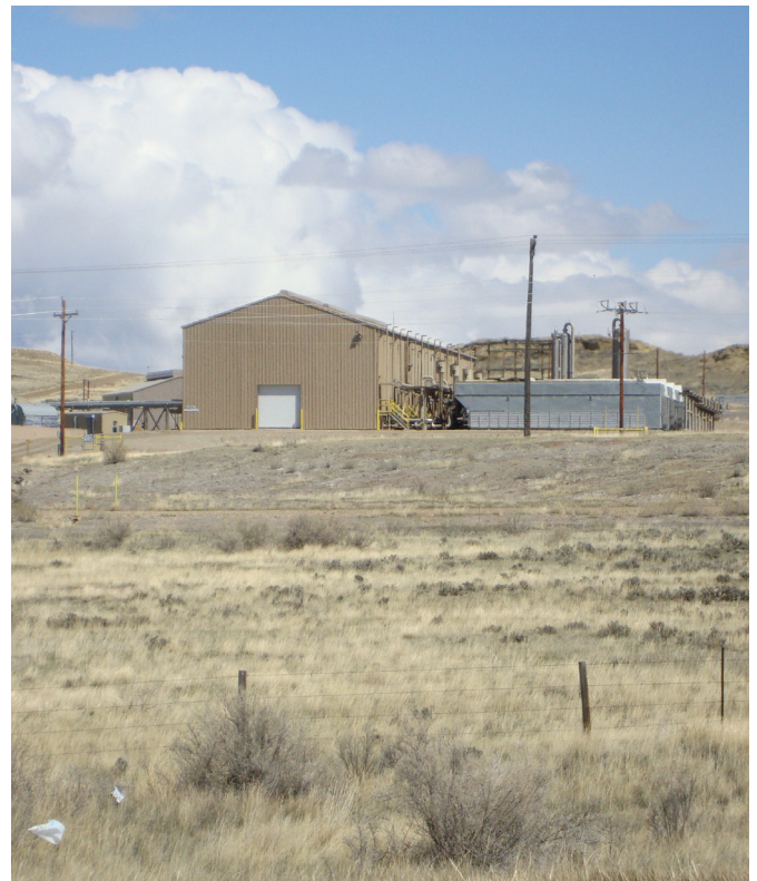
Salt Creek CO 2 Facilities
